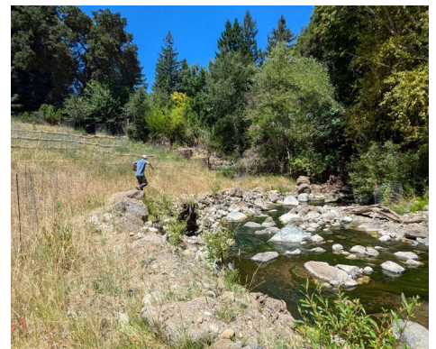
Private Emergency Creek Bank Repair, Portola Valley, California
