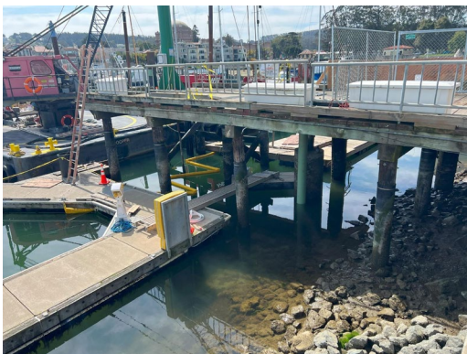
St. Francis Yacht Club Emergency Pier Repairs Project, San Francisco Bay, California.
